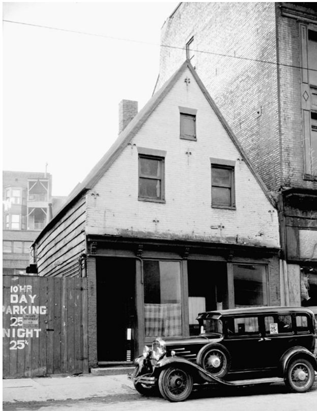
A late-17th- to early-18th-century Dutch gable home in Albany, New York, is typical of the Dutch architectural influence in the United States, with its Flemish brick bond and fleur-de-lis wall tiles. From the first Dutch settlements in the Americas in 1613, many villages were established by Dutch immigrants, including New Amsterdam, which eventually became New York City.
