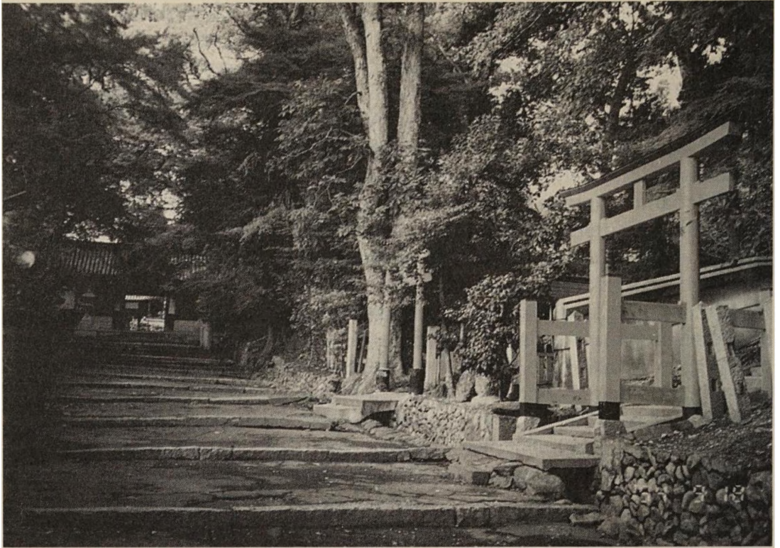
Torii marking the entry to the Inari chapel at Ikota Shrine. Photograph by Nakagawa Sugane.
